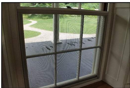
Above: screen insert installed in ballroom
