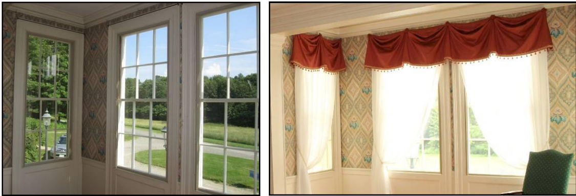
Interior storm windows installed
