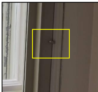
Above: Rivet pin installed to help secure side of storm window
