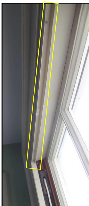
Left: Installation of U-channel at top of window casing
