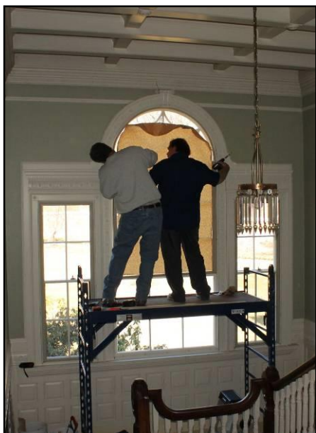
Installation of Palladian storm window
