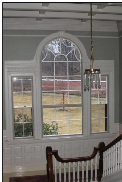
Palladian storm window installed
