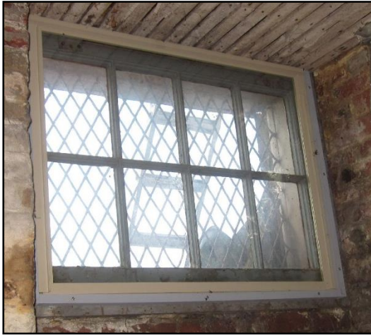
Basement window installation of storm window sash.
