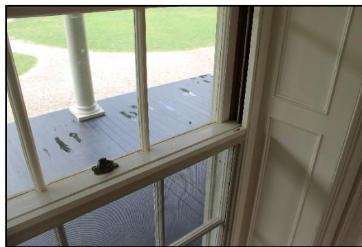
Above: Added support rail for screen / lower storm in ballroom
