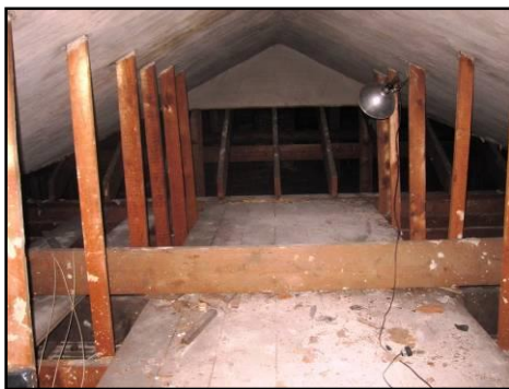
View of catwalk as seen from entry to ballroom attic space.
