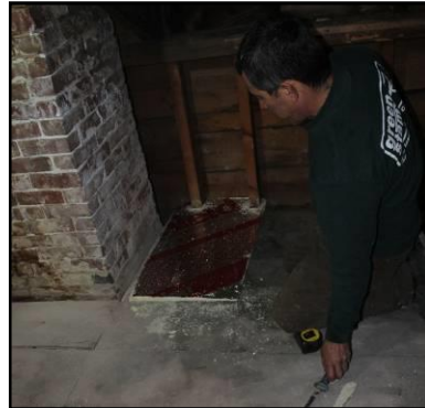
Foam board sealing around chimney chases
