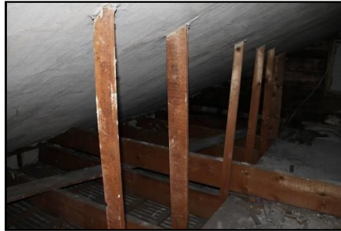
Catwalk space with open joist bays
