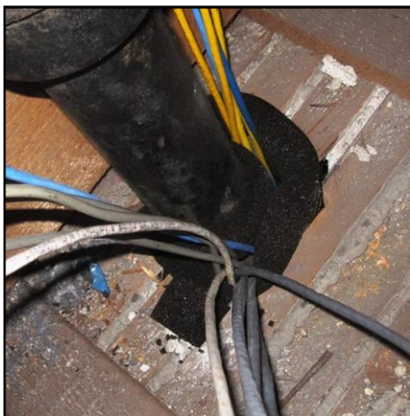
CC Expanding Sealer expands into opening created for plumbing and data cables
