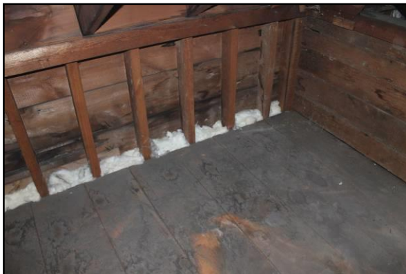
Roxul insulation fit into joist bay openings above the ballroom
