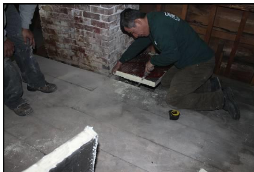
2" foam board cut to fit around opening adjacent to chimney above the ballroom
