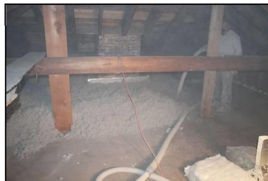
Filling the ballroom attic with insulation
