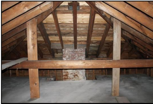
View over ballroom as seen from catwalk towards chimney at east end.
