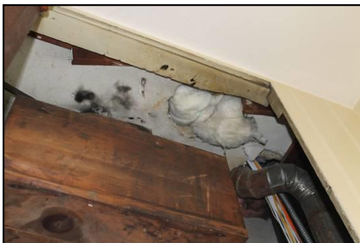
Roxul insulation fit into opening created by previous plumbing pipes
