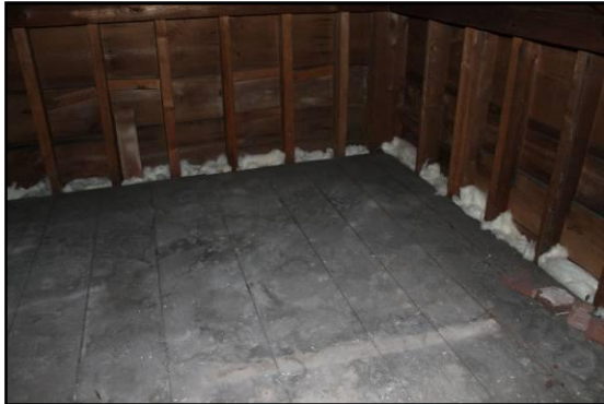
Insulation sealing the gaps in the wall pocket
