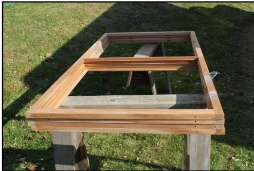
Storm window frames ready for dry fit to each opening
